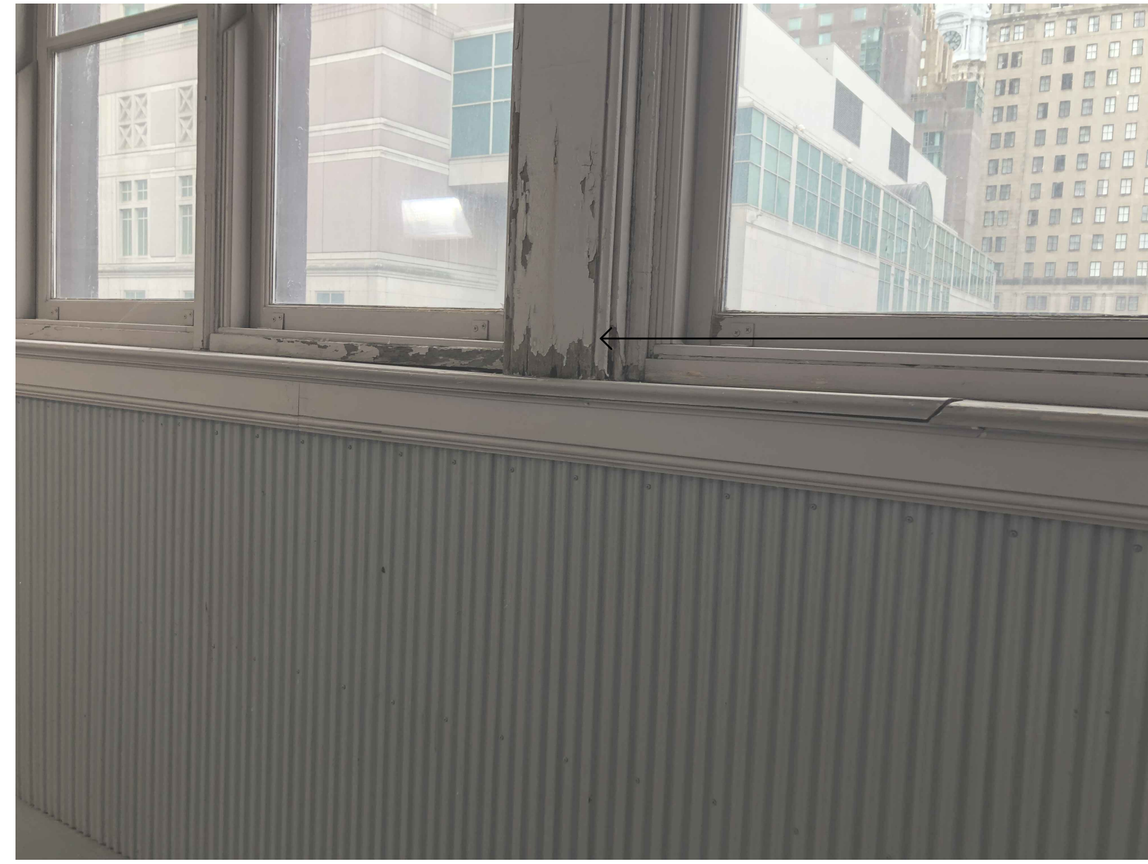
REMOVE AND REPLACE WOOD TRIM COMPONENTS
