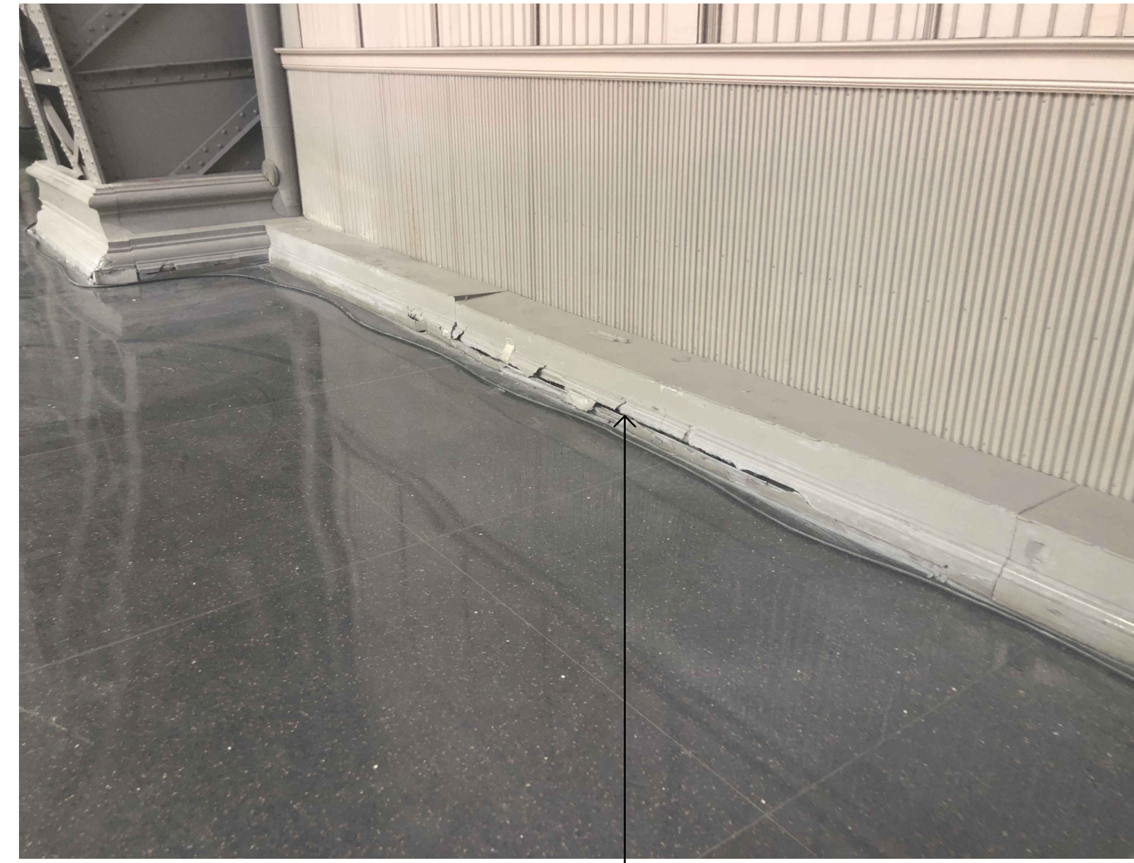
REMOVE AND REPLACE ALL GRFC BASE BETWEEN TRUSS 3 AND TRUSS 12
