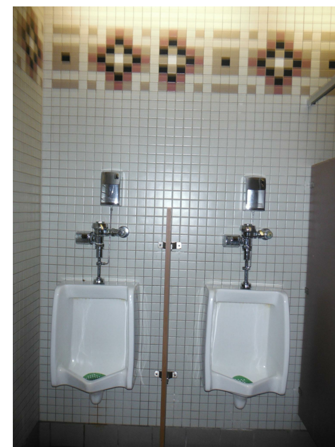
TYPICAL SMALL EXHIBIT RESTROOM - G MEN'S- EXISTING
