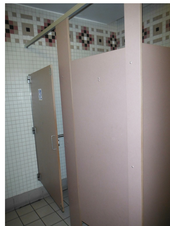
TYPICAL SMALL EXHIBIT RESTROOM - H MEN'S- EXISTING
