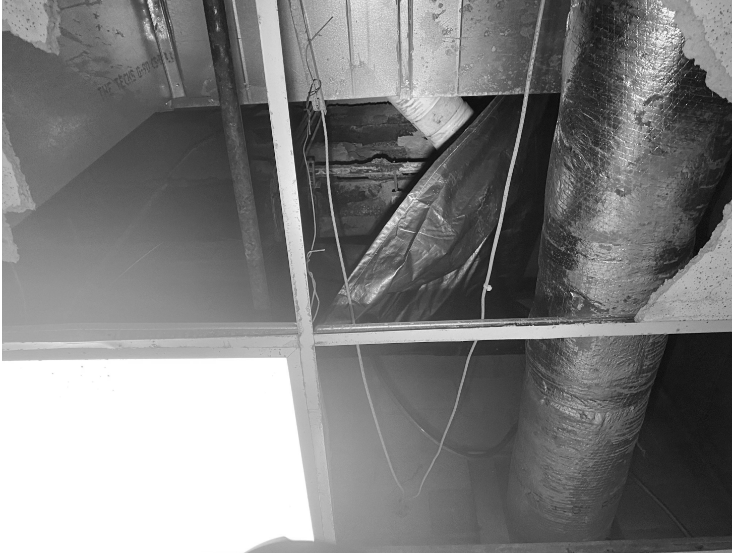
3 UNDERSIDE OF LOADING DOCK SLAB ON METAL DECK SCALE: 12" = 1'-0"
