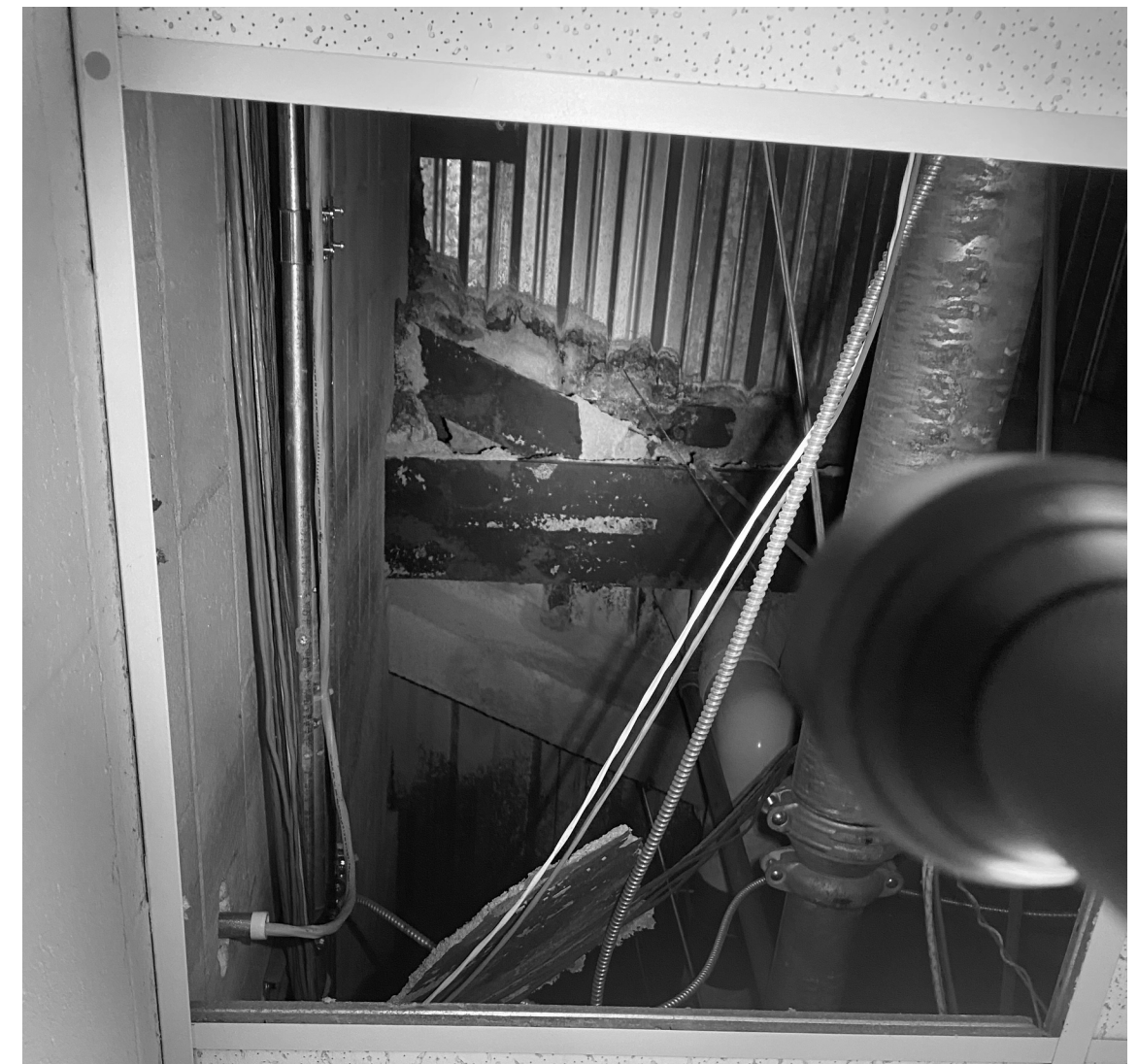
2 UNDERSIDE OF LOADING DOCK SLAB ON METAL DECK SCALE: 12" = 1'-0"
